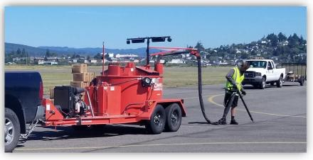
grow, which can cause more damage over time. Equipment was used that grinded out all excess dirt and vegetation within the cracks. Then a special sealant was used to fill in any of those areas. By addressing this issue early on, the airfield pavement will maintain its structural integrity for many years to come.
