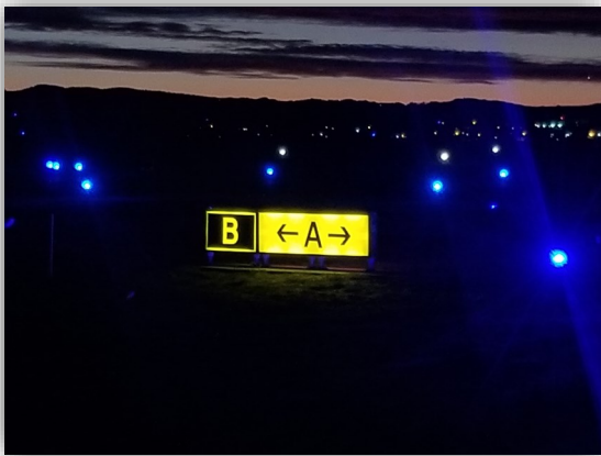
Newly upgraded taxiway and sign lighting
